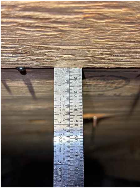
7/16" Plywood/OSB Roof Sheathing
